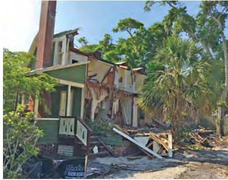
405 S Osprey being demolished
